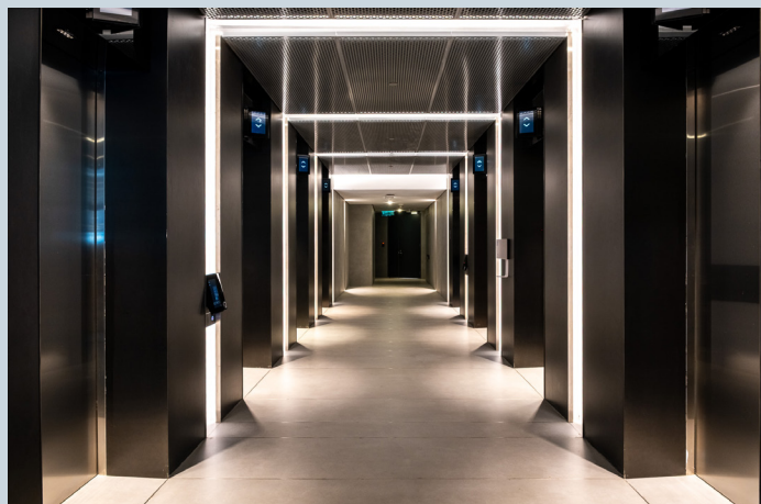
Photo of a lift lobby at a typical office floor in the tower (courtesy of PMV). Note the e-displays functioning as conventional hall lanterns, combined with numeric keypad hall stations.
